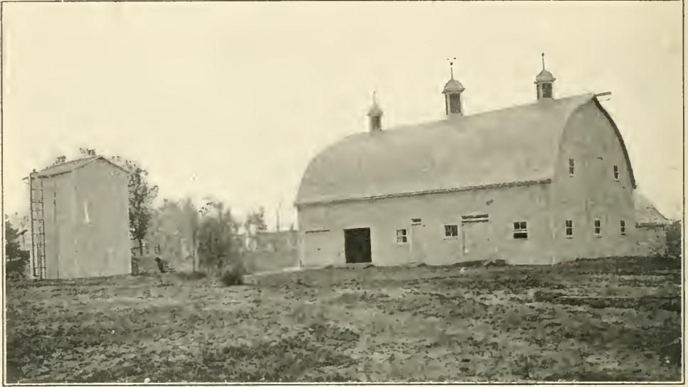
Barn and Ice Cold Storage House.
